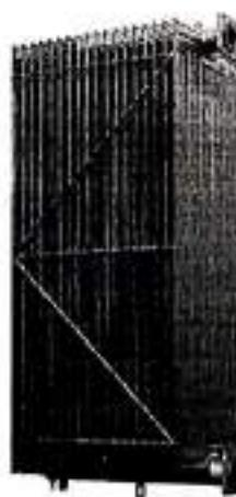
The transformer is made up of exterior radiator tubes, which are cooled by air from fans installed on the tank's walls. Most of the time, heat is produced as a result of the power that is lost in the transformer. Most dry transformers use natural air cooling.
